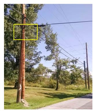
A. <u>Dangerous Double Poles.</u> The picture at left from Chester County shows two sets of double poles (one in the foreground and one in the background). The old pole in the foreground is clearly marked with an "X" indicating it is to be removed. This pole is so bent that it is tied to the new pole at the top to keep it from falling over (see blow-up below of area outlined in yellow). It appears that VZPA's facilities are the only ones still attached to the old poles.
