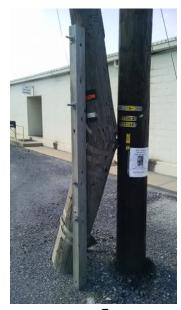
E. Old double poles can become so bent that they require supports to try to keep them upright. The picture at right from Berks County shows a seriously bent old double pole.
