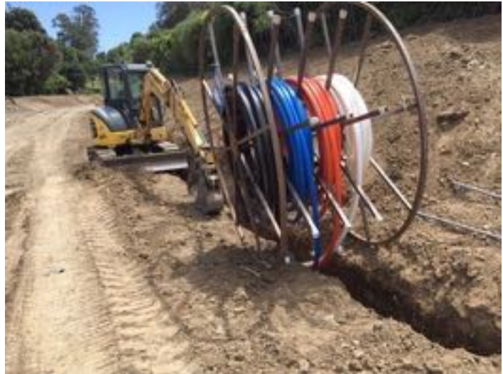
Figure 2.2 – Fiber optic conduit.
