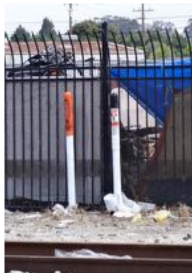
Figure 3.2 – Fiber route markers on Union Pacific right of way in downtown Salinas.
