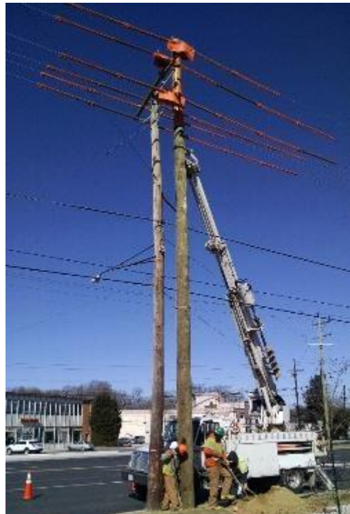
Figure 12: OSP Crew Replacing a Pole
