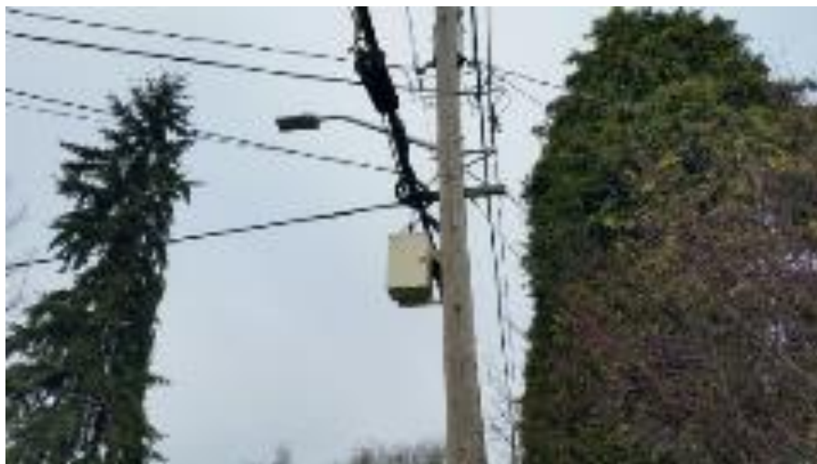
Figure 20: Example Small Outdoor FDC Housing PON Splitters
