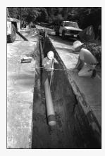
Backfilling the trench and compacting the fill in layers
