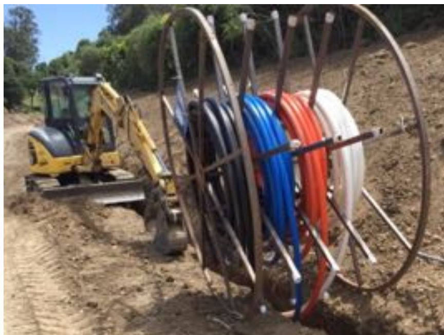
Dig once, open trench, shadow conduit policies in Sonoma, Brentwood, Salinas
