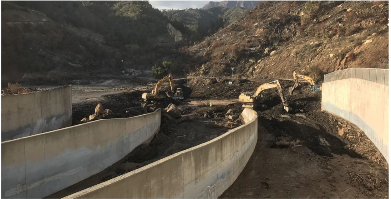
5 6 7 8 9 10 11 12 13 14 15 Figure 6 - Santa Monica Creek Debris Basin
