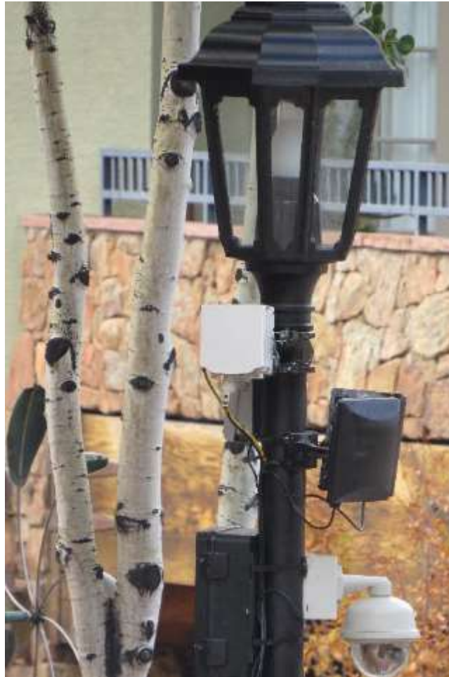
Figure 8 – mmWave Antennas Providing Backhaul for Wi-Fi Network
