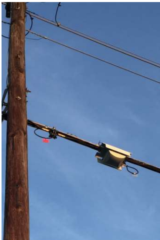
Figure 9 – Wi-Fi Antenna on Cable TV Attachment
