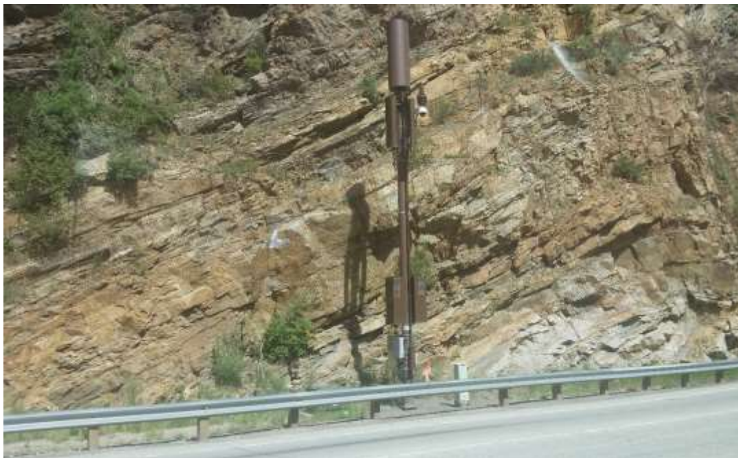
Figure 11 – Distributed Antenna Installation on U.S. Route 6 in Clear Creek County, Colorado
