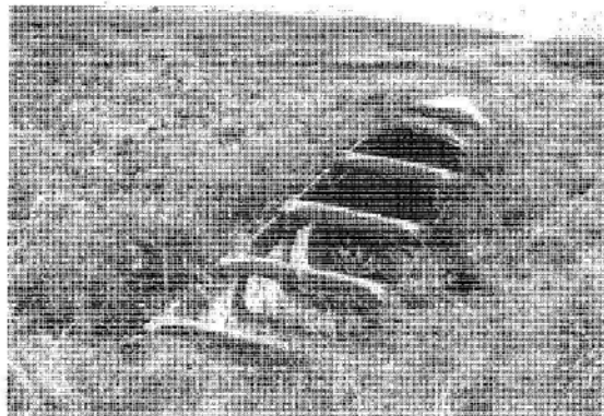
Figure 3-12. Safety Treatment for Parallel Drainage Pipe
