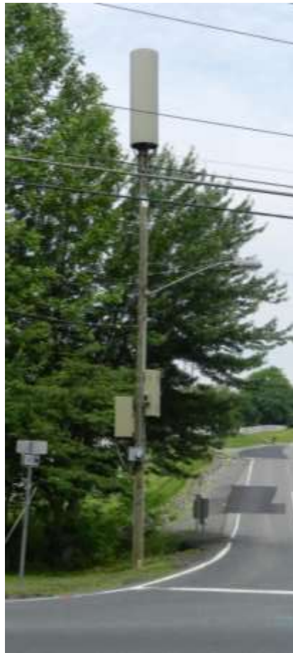
Figure 2 – Multifrequency DAS Structure with Multiple DAS Antennas
