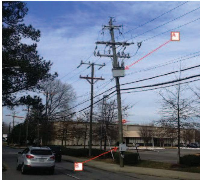
Small wireless facilities are consistent with such existing installations, as the next photograph of a Crown Castle node in Newport News demonstrates. Crown Castle's node is on the pole on the left side of the road, across from the line of poles that are of equivalent height. Indeed, at least one of those other poles has a group of large electric transformers.
