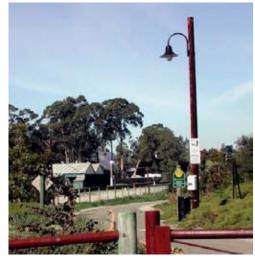
Trail lighting that is Dark sky compliant due to downward facing light with shield
