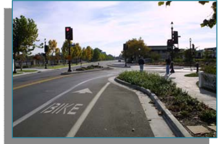
Example of geometric and landscaping features intended to reduce motorist speed at a roundabout.
