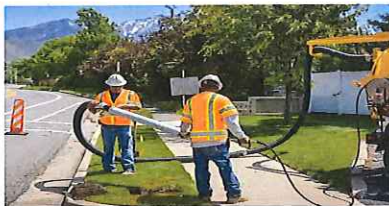
Safety is always a huge concern for us. By using a vacuum and potholing equipment to locate existing utilities, we can work around important infrastructure as we lay our fiber.
