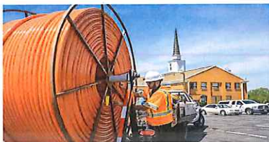
This bright orange roll of conduit covers our fiber to protect it from the elements as we lay it underground. We'll be installing enough fiber in Salt Lake City to run from here to Canada.
