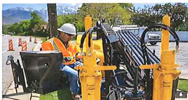
We use a lot of different types of equipment to lay fiber. Here we're preparing the horizontal directional drill to place conduit underground.
