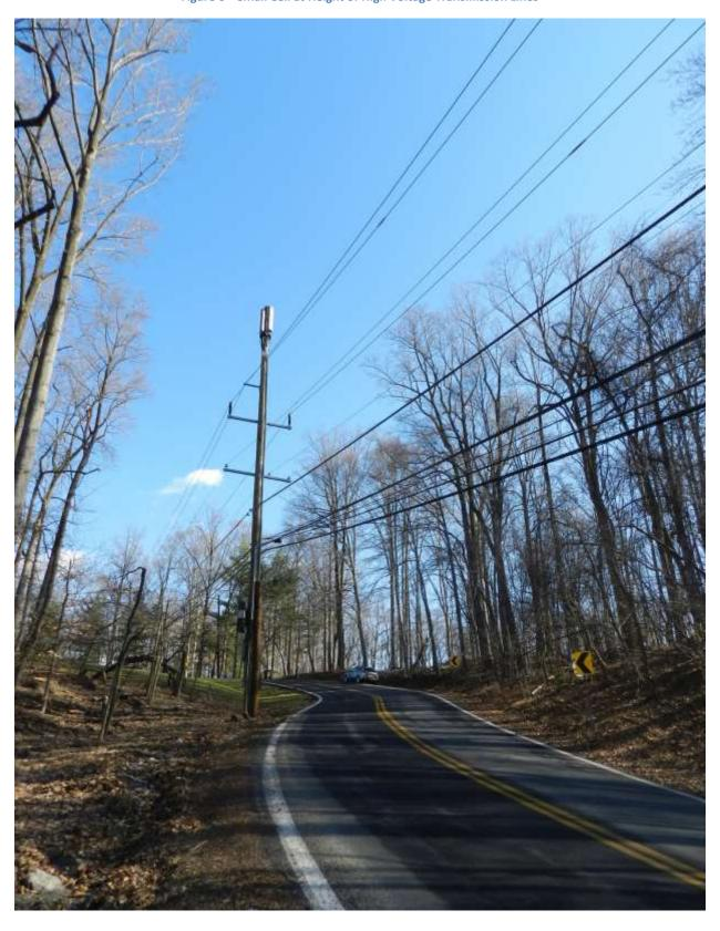
Figure 6—Small Cell at Height of High Voltage Transmission Lines
