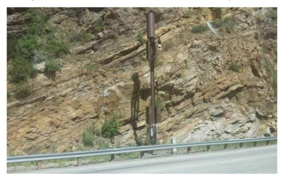
Figure 11 – Distributed Antenna Installation on U.S. Route 6 in Clear Creek County, Colorado
