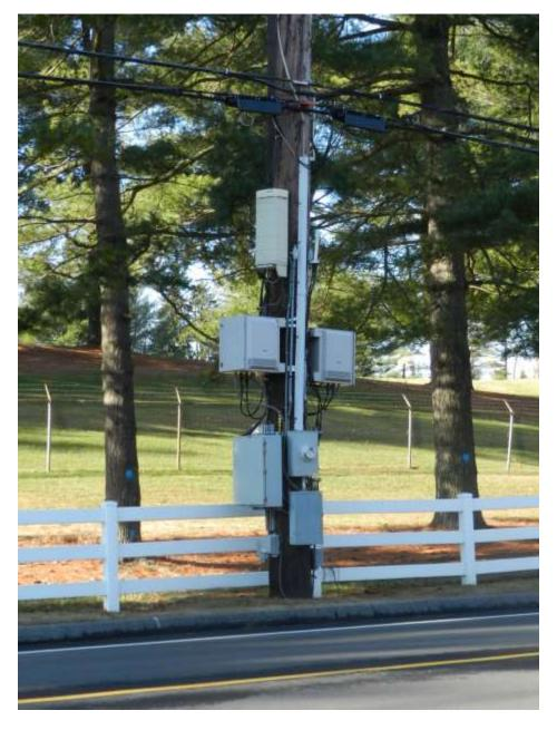
Figure 4 – Base of DAS Installation With Multiple Cabinets for Radios, Backhaul, and Power
