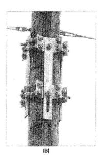
Figure 4-14. Prototype Breakaway Design for Utility Poles
