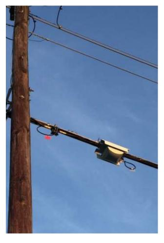
Figure 9 – Wi-Fi Antenna on Cable TV Attachment
