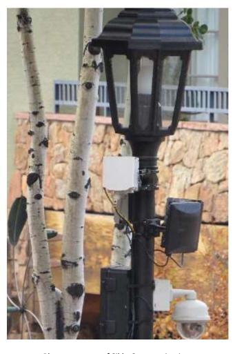
Figure 8 – mmWave Antennas Providing Backhaul for Wi-Fi Network
