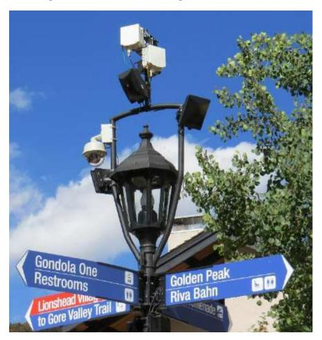
Figure 7 – mmWave Antennas Providing Backhaul for Wi-Fi Network
