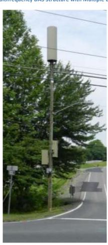
Figure 2 – Multifrequency DAS Structure with Multiple DAS Antennas
