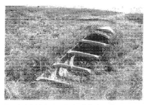
Figure 3-12. Safety Treatment for Parallel Drainage Pipe
