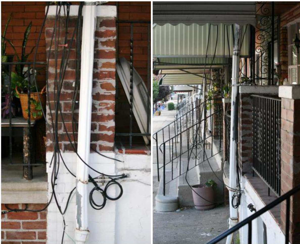
Picture 9. [REDACTED] – Cable drop is not properly attached to building creating an entanglement potential and it is aesthetically problematic. (Comcast states: Fixed, removed unused drop and ran new drop and properly attached to the house. 6/19/2014).
