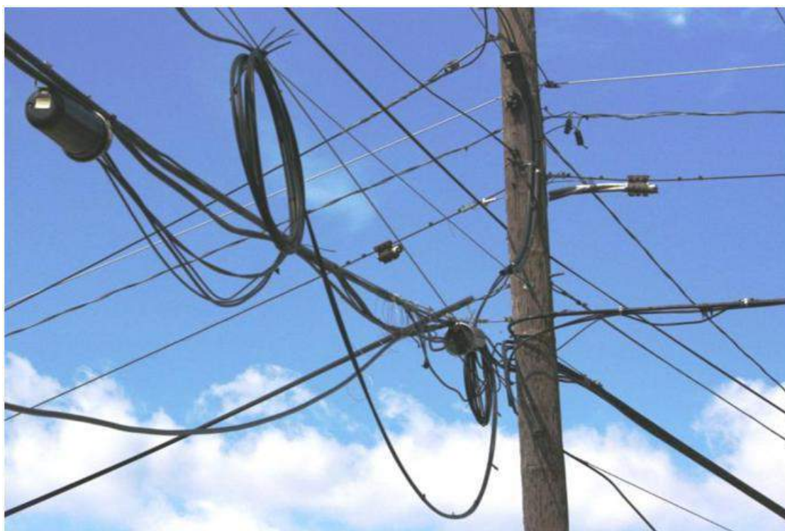
Picture 13 and 14. 56th St & Lindbergh Blvd – Lashing wire is broken and cables are hanging down from strand. (Comcast's response: De-lash, re-lash complete. 6/30/2014)
