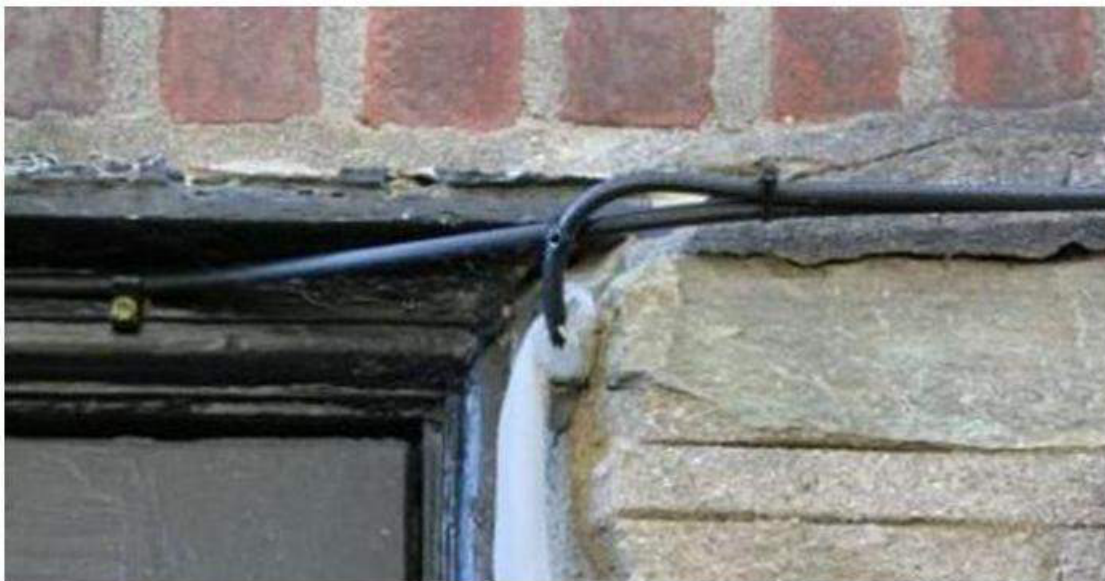
Picture 3. [REDACTED] – Cable goes directly into building. No visible ground/bond on drop and no tag to indicate ground/bond inside. (Comcast states: Fixed, grounded drop to adhere to BRIS [Comcast's Broadband Residential Installations Standards] Standard. 6/18/2014)
