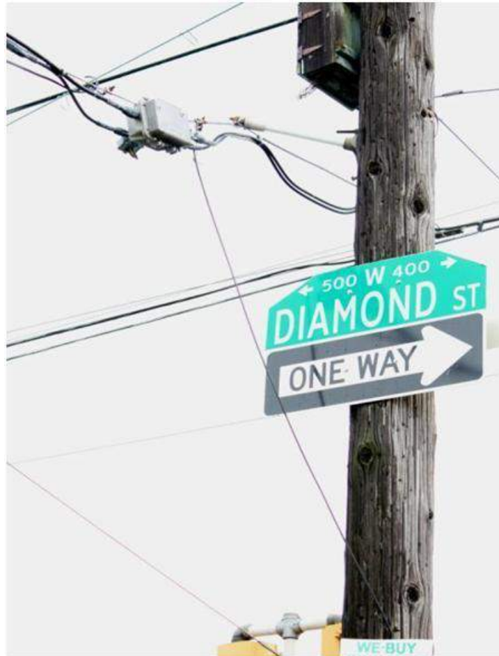
Picture 6. Diamond St W & 5 th St N – Drop not properly attached to pole – hangs out from pole creating a problem for workers climbing the pole. (Comcast states: Re-Jack strand, re-spliced strand, re-sag – completed 6/25/2014).)
