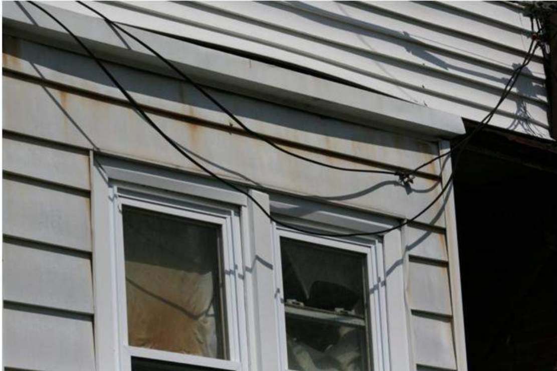
Picture 8. [REDACTED] – Drop is not properly attached to the building. Drop is hanging in front of a window. (Comcast states: Not active, knocked on door and called customer with no answer. Common ground inside. 6/18/2014). NOTE: Explanation from Comcast doesn't match violation found.
