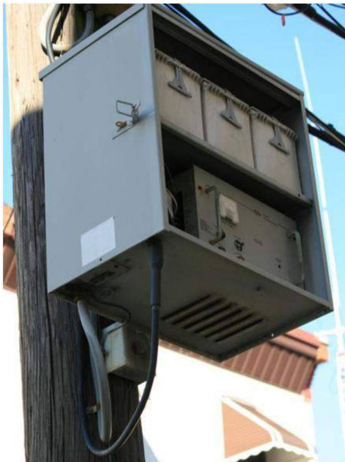
Picture 15. 1607 N Cadwallader St – Power supply and breaker box are not locked. Box cover is missing. (Comcast’s response: Power supply removed. 6/20/2014)
