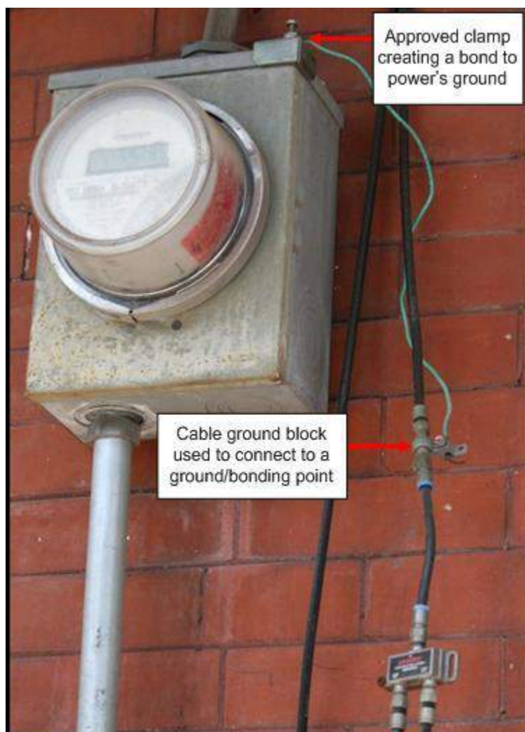
Picture 2. [REDACTED] - Proper bond - Bonding wire comes from Comcast's ground block and attaches to the metal meter box with an approved clamp. (Cable and ground wire though need better attachment to the building)
