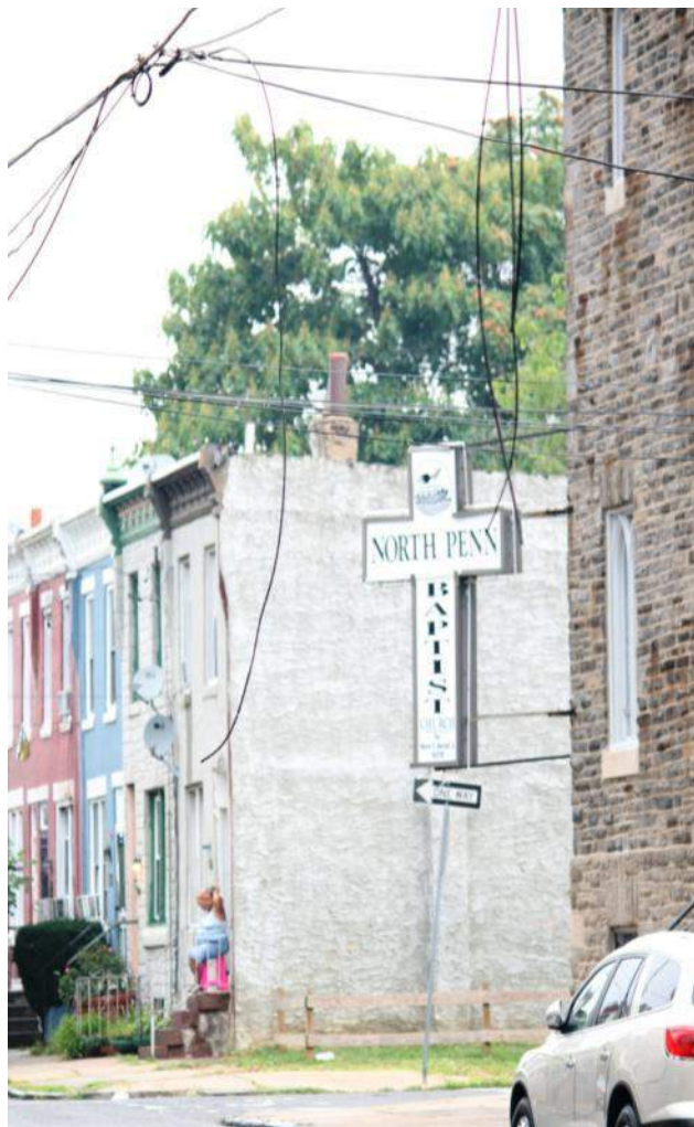
Picture 7. 2411 N 27 th Street – Cables hanging down from strand only 6-7 feet above ground. (Comcast states: Fixed, removed 4 drops 6/18/2014)
