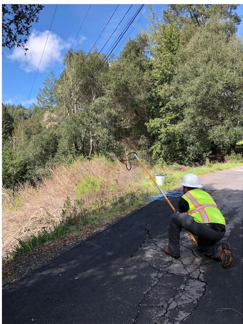
*Figure 3 – Contractor launching throwline for a fiber pull in the CASF Nicasio Broadband Project, Western Marin County.*
