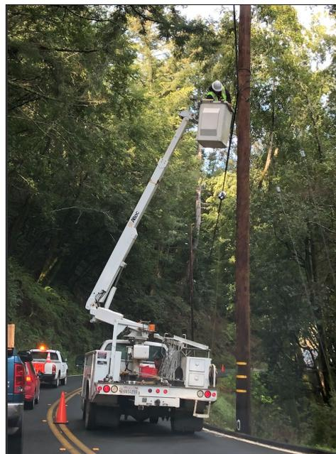
*Figure 2 – Aerial fiber installation to provide broadband service in the CASF Nicasio Broadband Project, Western Marin County.*
