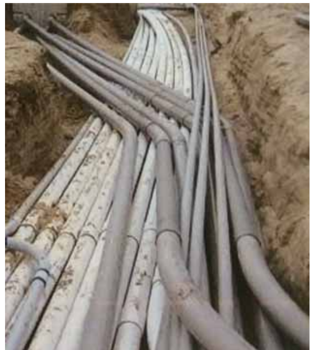
Figure 7.2 – Conduit in Bridge district joint trench. Photo credit: City of West Sacramento.
