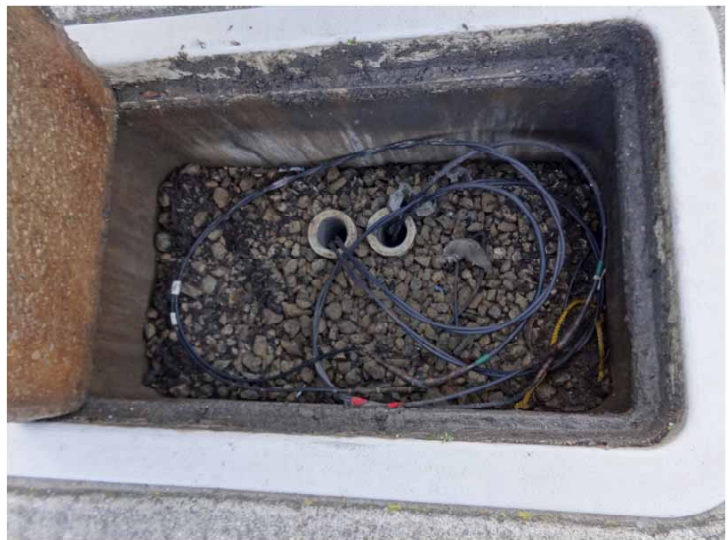
Figure 4.2 – Traffic signal interconnect system hand hole.
