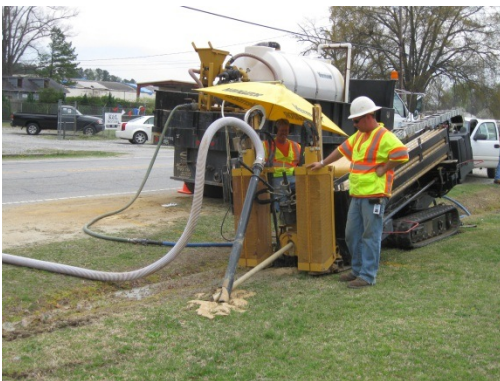
A worker installs subterranean conduit and fiber.
