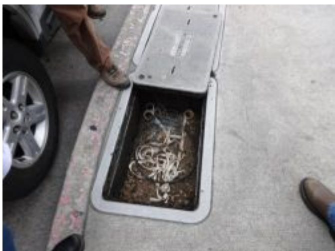
Figure 4.1 – City-owned telecommunications conduit, installed by Comcast in downtown area.
