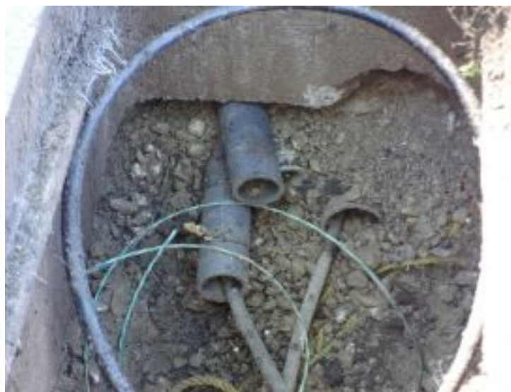
Figure 4.2 – City of Berkeley conduit.
