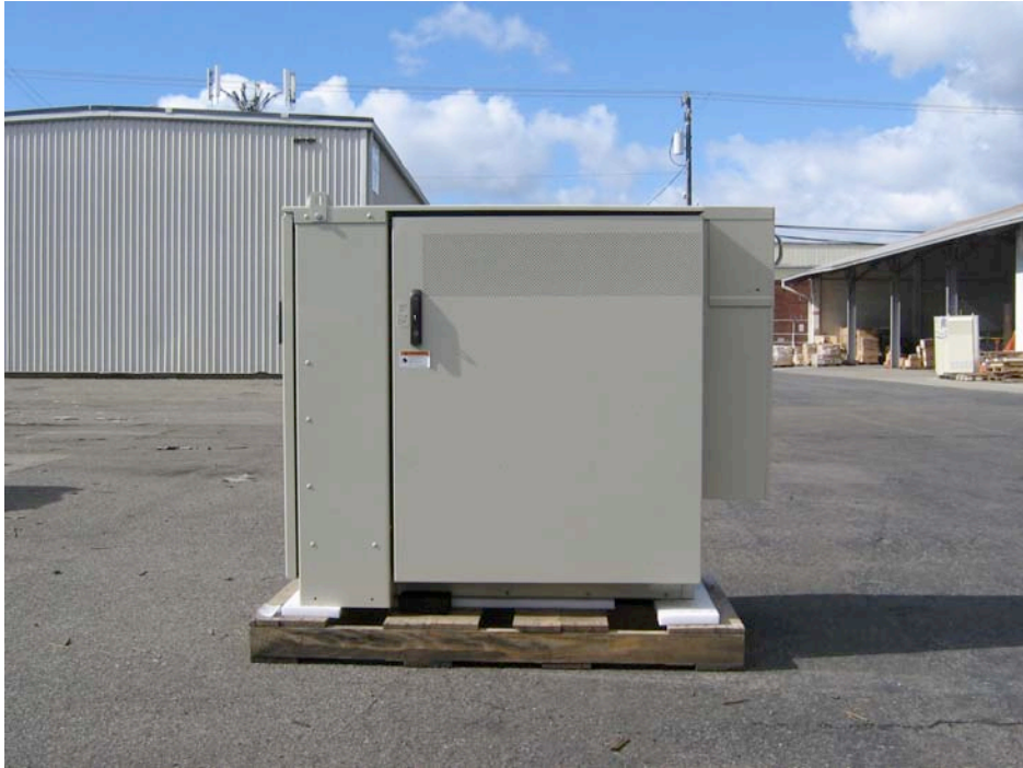
Typical utility box installation for Project Lightspeed
