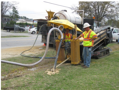
A worker installs subterranean conduit and fiber.
