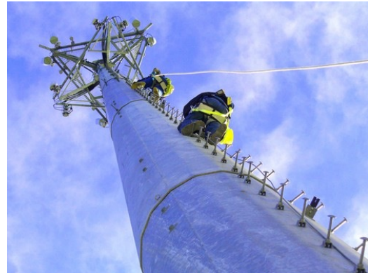
Unified communications: Fiber and Cellular networks are one in the same
